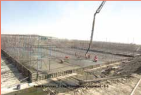
Raft concreting completed at E3 roads in Activation Area
