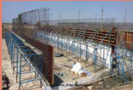
Construction of Bridge in Activation Area
