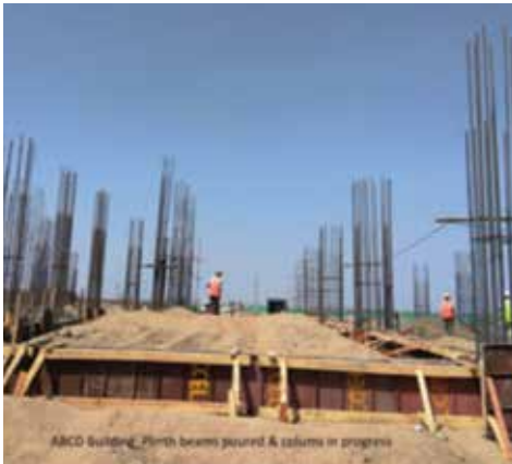
Construction of Plinth beams poured and column in progress
