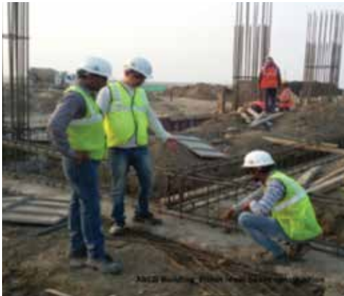
Construction of Plinth level beams
